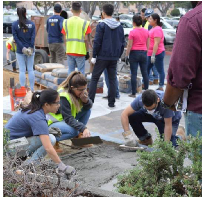
CONSTRUCTION COMPETITION Members paving the concrete sidewalk during the competition
